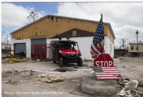
Fire Station Just After the Storm
