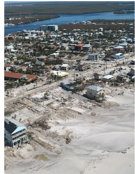
Damages to the Town as Pictured from an Aerial Tour Conducted by the County with Hagerty
