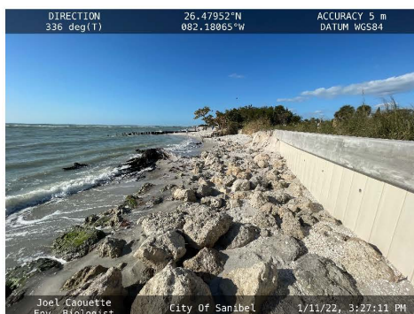
Photo 3. Site conditions on 1/11/22 looking northwest
