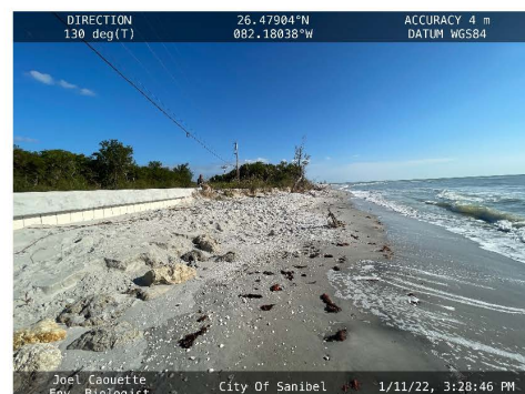
Photo 4. Site conditions on 1/11/22 looking southeast
