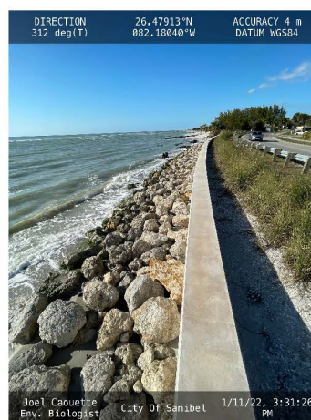
Photo 5. Site conditions on 1/11/22 looking northwest
