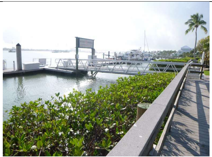
4. View of Mangroves, facing north
