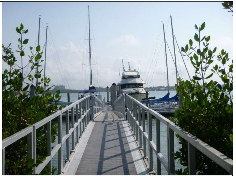
32. View of access walkway facing northeast
