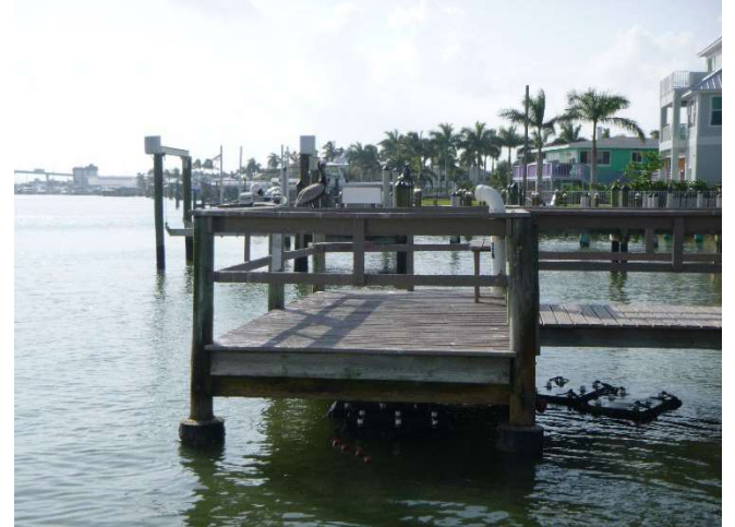
24. View of terminal platform, facing south
