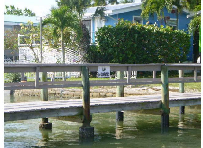
23. View of no mooring signs, facing south
