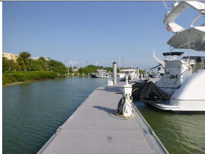
12. View of terminal platform facing North
