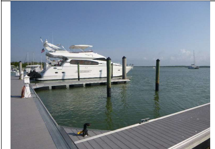
11. View of wrapped pilings
