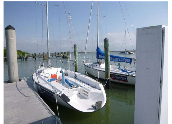
36. View of finger pier facing north
