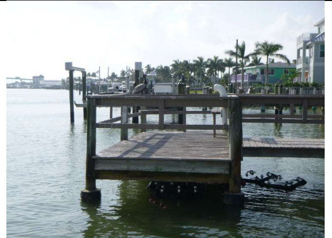
24. View of terminal platform, facing south
