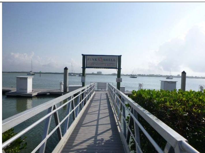
8. View of access walkway facing northeast
