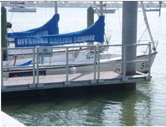
33. View of finger pier and no mooring signs facing northeast
