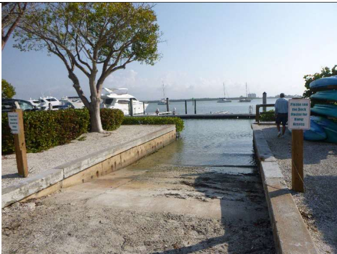
3. View of Kayak launch, facing northeast
