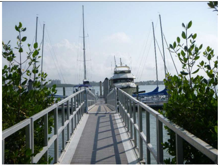
32. View of access walkway facing northeast
