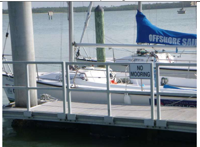
34. View of finger pier and no mooring signs
