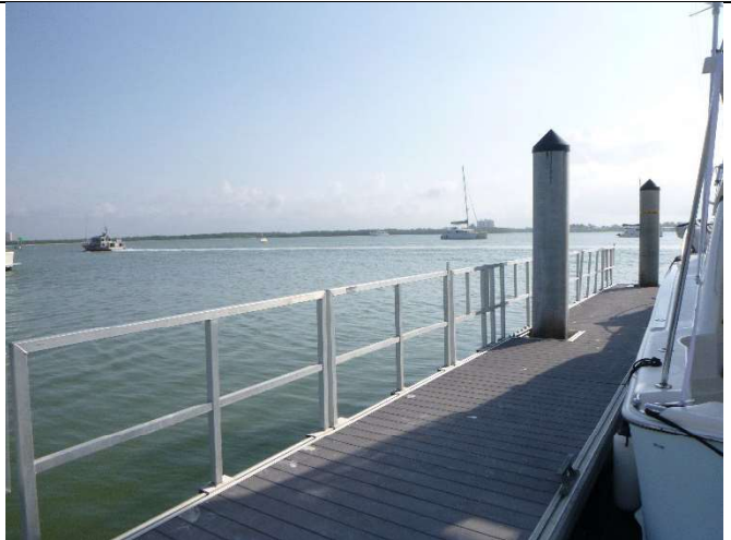
16. View of finger pier facing northeast
