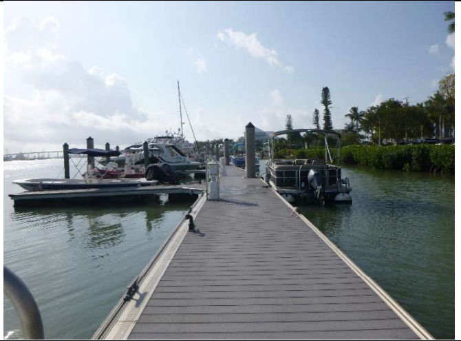
18. View of terminal platform facing south
