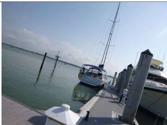
37. View of dock facing east
