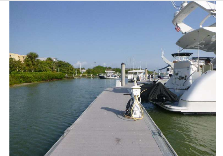
12. View of terminal platform facing North
