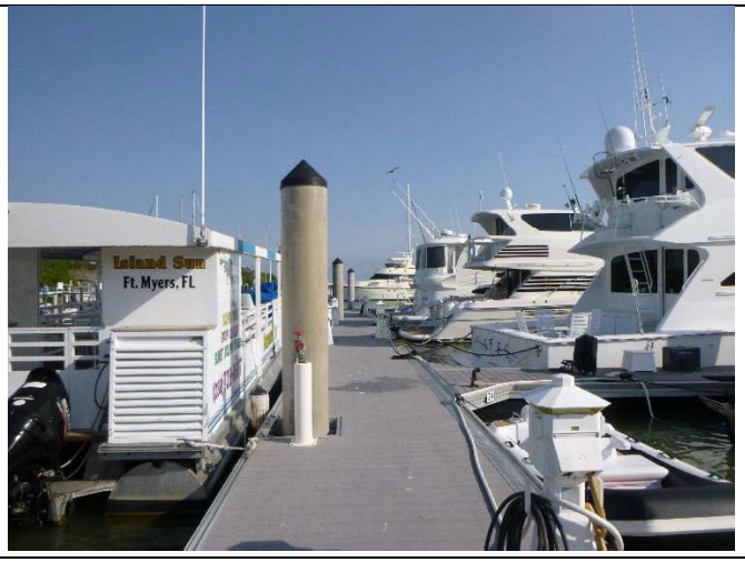
14. View of terminal platform and slips facing North
