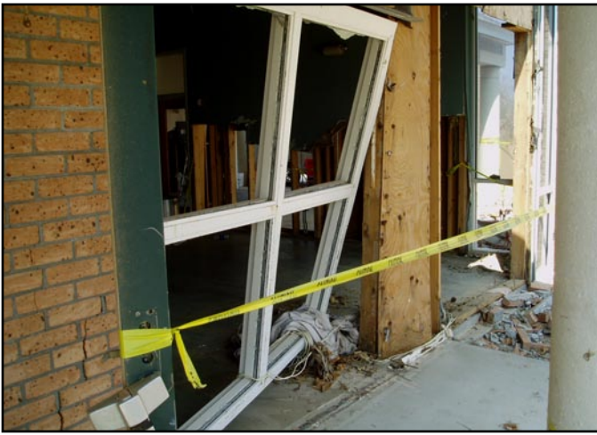
Figure 3. Failure of wood-frame wall, brick veneer, and windows as a result of 4 feet of stillwater flooding and small waves (Hurricane Katrina).
