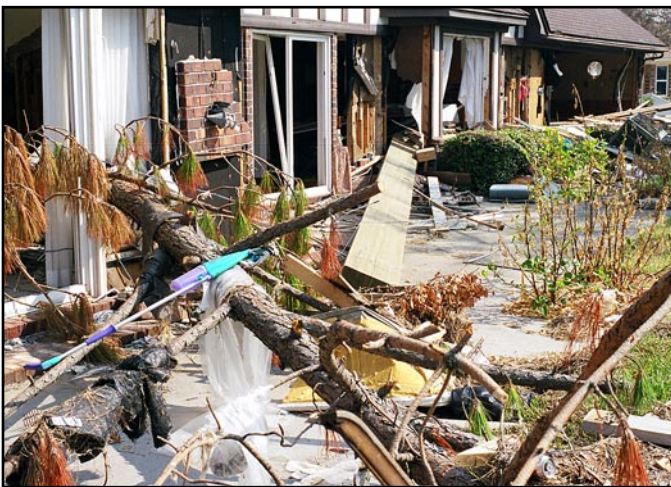
Figure 5. Damage to light frame walls due to floating debris and small waves. The damaged home was in the third row back from a bay shoreline (Hurricane Ivan).
