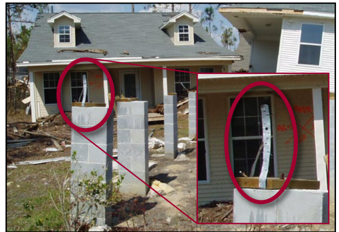
Figure 8. Post-Katrina investigations showed that many buildings were attached to foundation piers with light gauge metal straps. These straps failed in many instances. A stronger (preferably bolted) connection is recommended when attaching Coastal A Zone buildings to their foundations.
