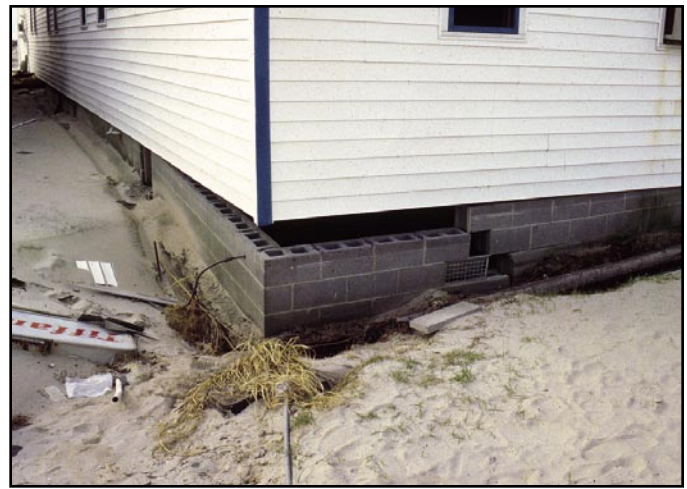
Figure 4. Failure of A Zone type foundation in coastal area, not subject to V Zone conditions (Hurricane Fran).
