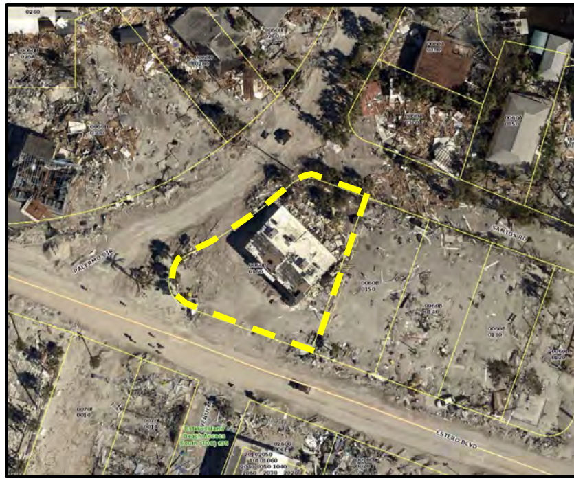
Figure 3. Post Hurricane Ian
