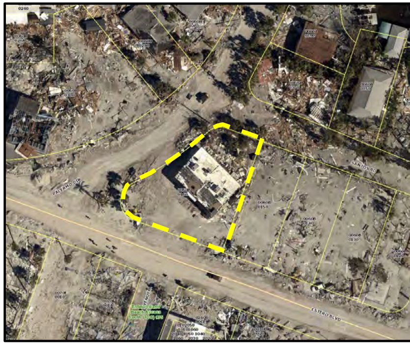
Figure 3. Post Hurricane Ian
