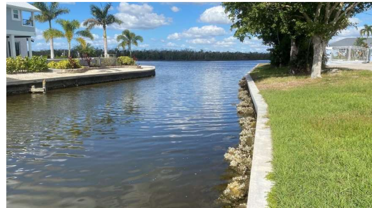
Figure 4-23. Seawall at Fort Myers Beach
