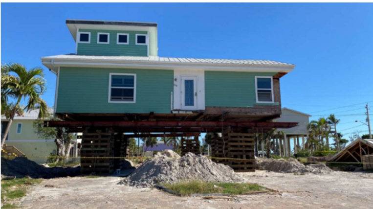
Figure 2-1. Elevating a Housing Unit
