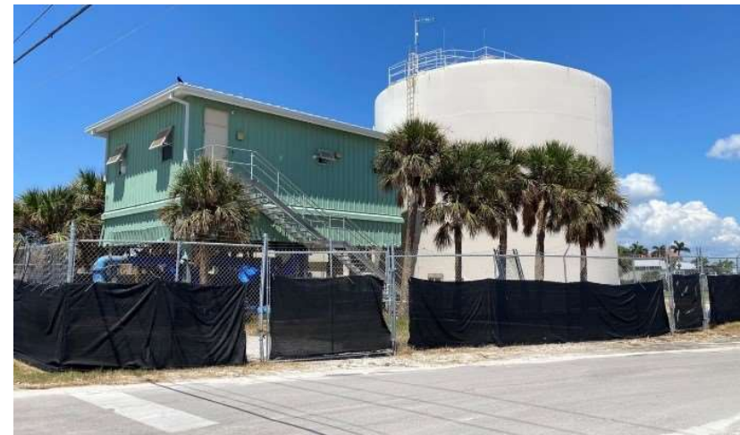
Figure 4-24. Water Supply Tank and Pump Facility
