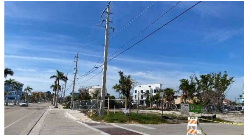
Figure 4-25. Above-ground Utility Lines
