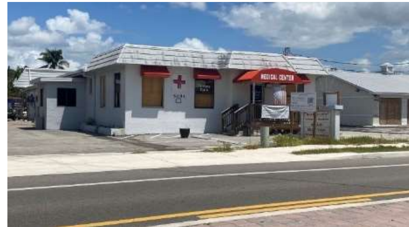
Figure 4-27. Former Urgent Care Medical Facility at Fort Myers Beach
