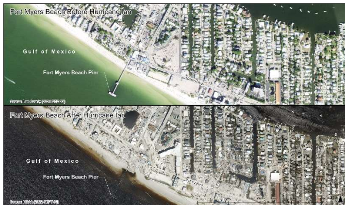
Figure 3-18. Aerial Imagery of the Fort Myers Beach Pier and Times Square Before and After Hurricane Ian
