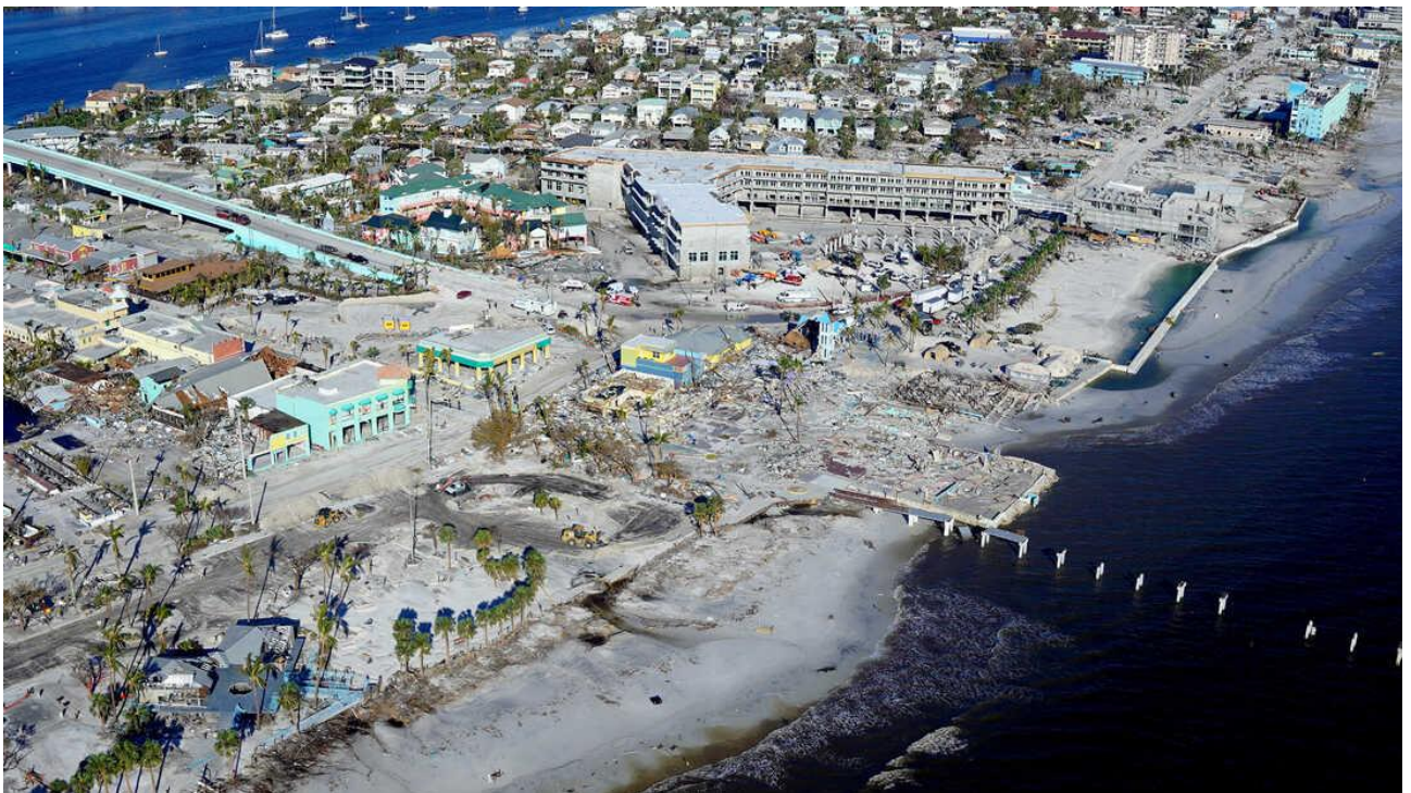
Figure 6. Hurricane Ian Damage on North Estero Island.
