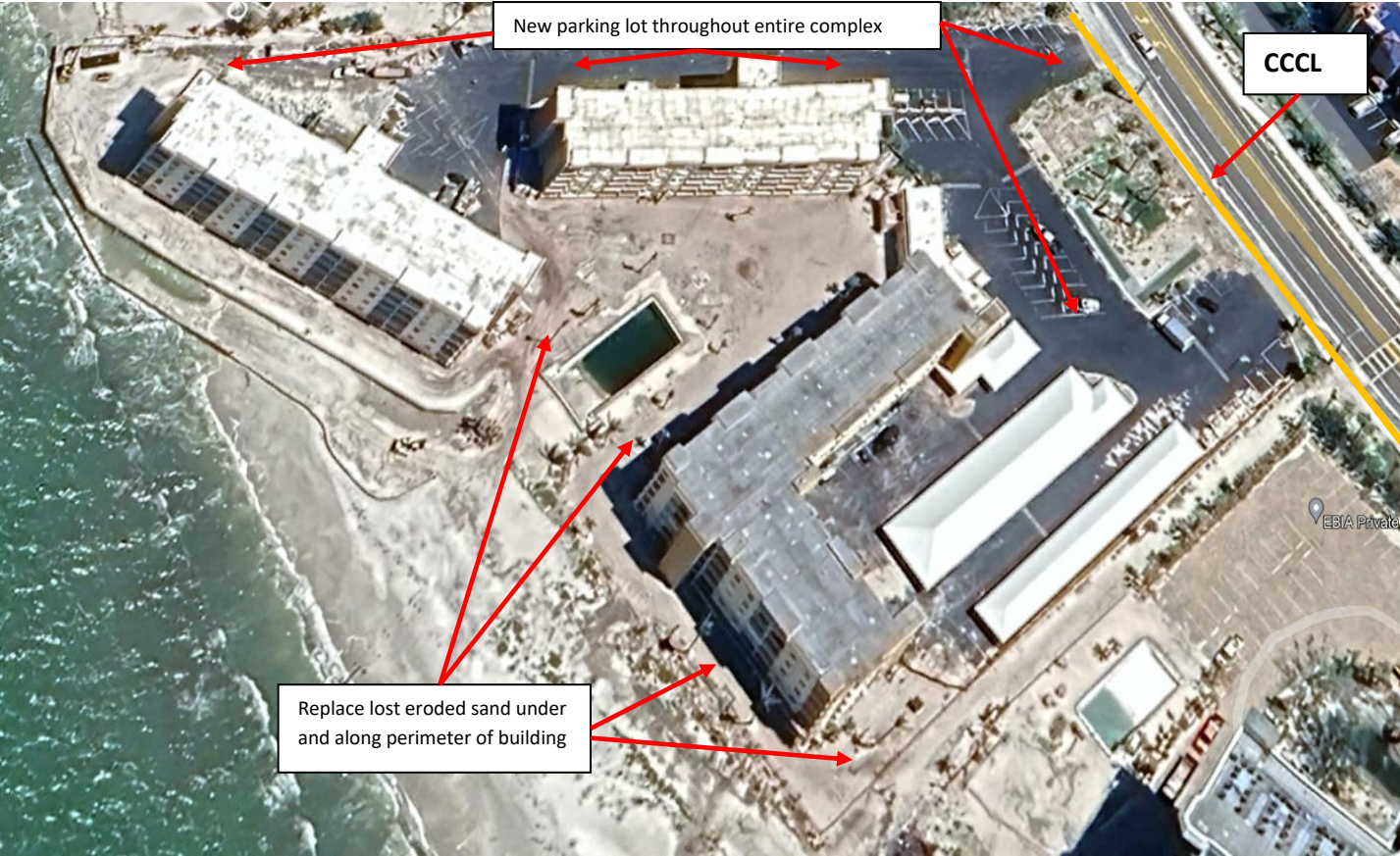
Leonardo Arms Complex After Hurricane Ian With Retaining Wall Under Construction.
