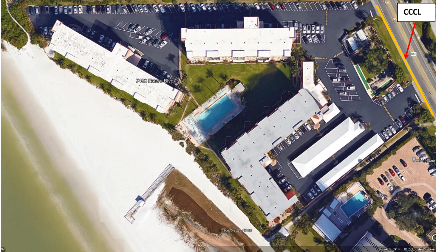
Leonardo Arms Complex Before Hurricane Ian
