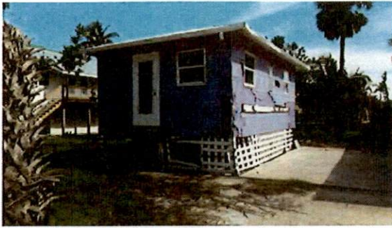
Building Front Photo
