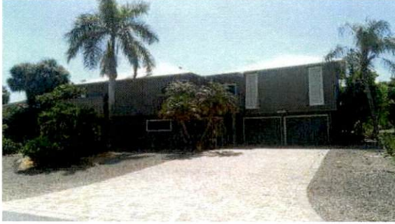
Building Front Photo
