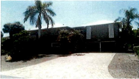
Building Front Photo
