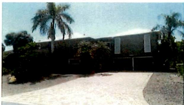
Building Front Photo
