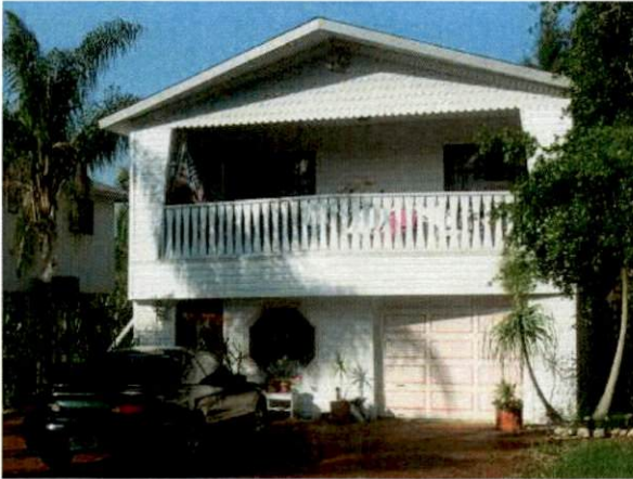
Building Front Photo
