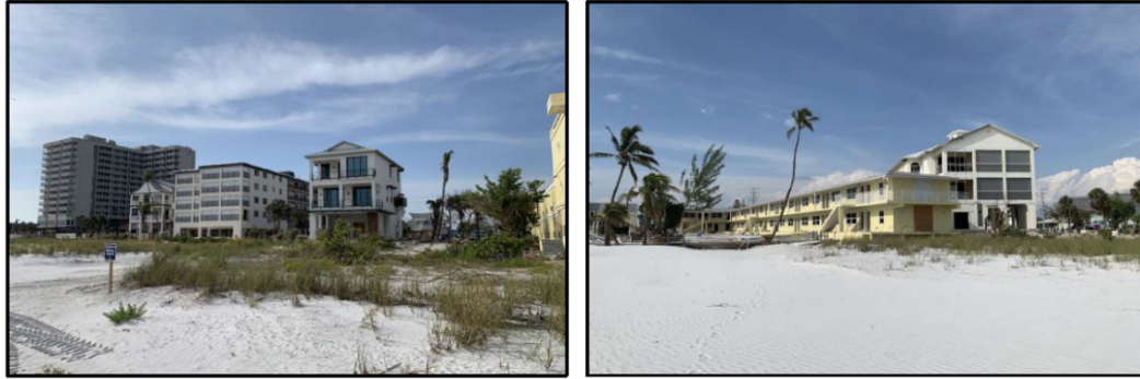
Figure 2. Photos of adjacent building heights. (West – left and East – right)
