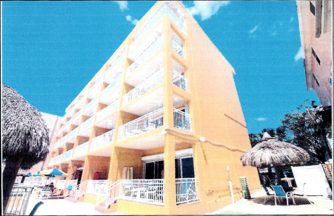
EXTERIOR VIEW OF RESIDENTIAL BUILDING
