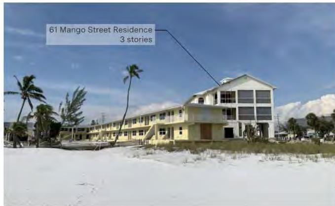
east context building
