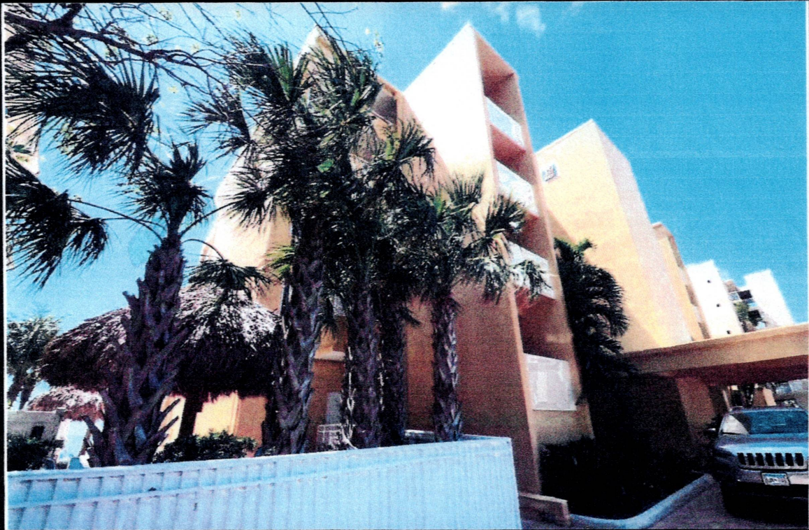
EXTERIOR VIEW OF RESIDENTIAL BUILDING
