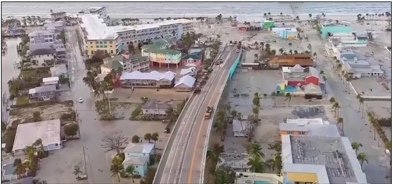
Figure 9. Hurricane Milton Damage on North Estero Island.
