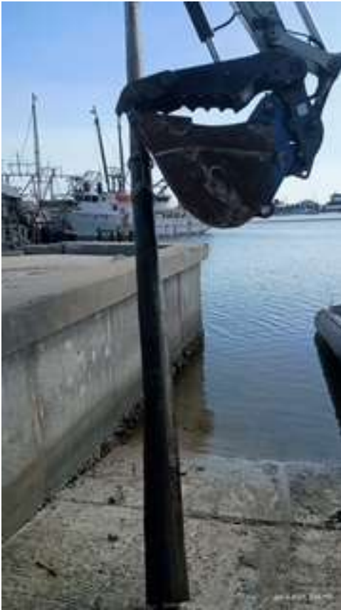
1/7/2025 EASTWALL 3 RD PILING
