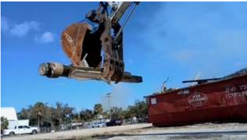
1/7/2025 EASTWALL PILING / ROPE
