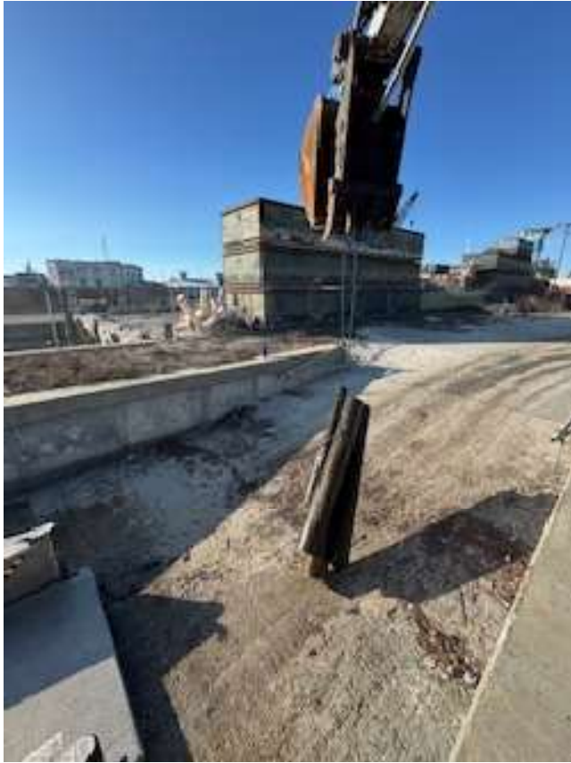
1/7/2025 EAST WALL NORTH PILING
