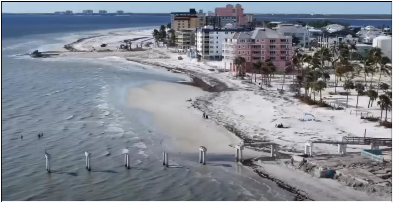
Figure 6. Hurricane Helene Damage on North Estero Island.
