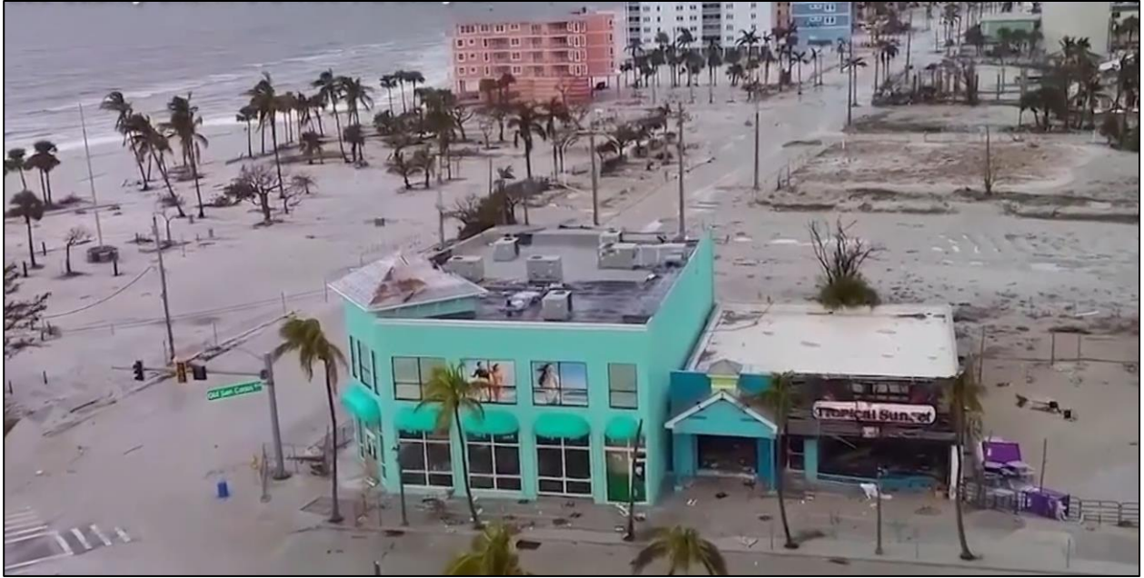
Figure 8. Hurricane Milton Damage on North Estero Island.
