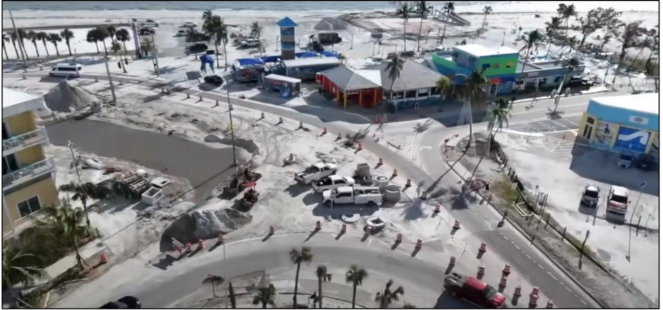
Figure 7. Hurricane Helene Damage on North Estero Island.
