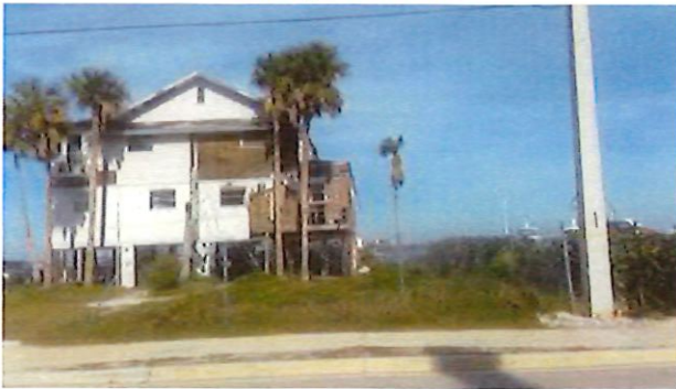
Building Front Photo
