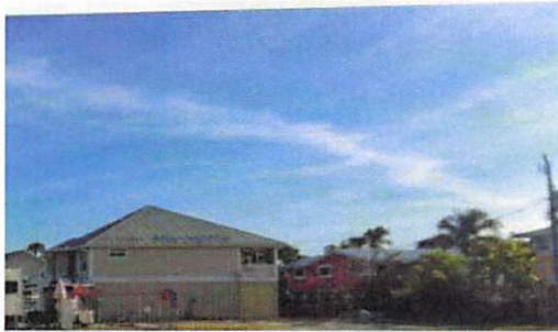
Building Front Photo
