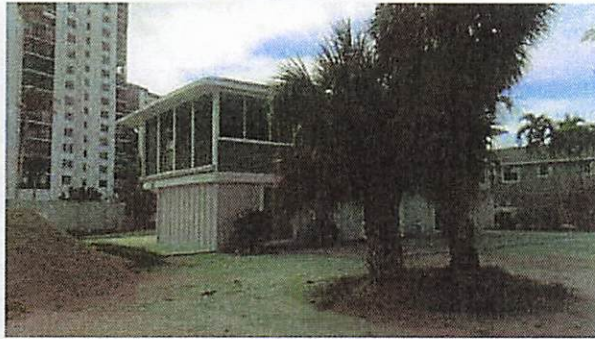
Building Front Photo
