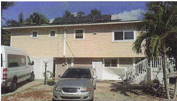
Building Front Photo
