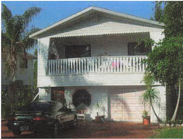
Building Front Photo
