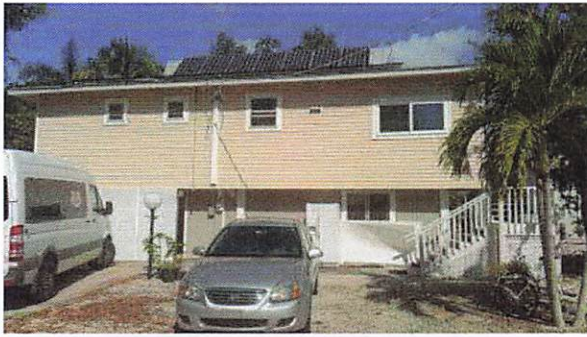
Building Front Photo
