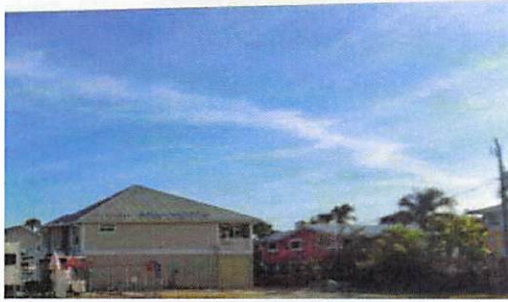
Building Front Photo
