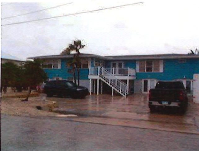
Building Front Photo
