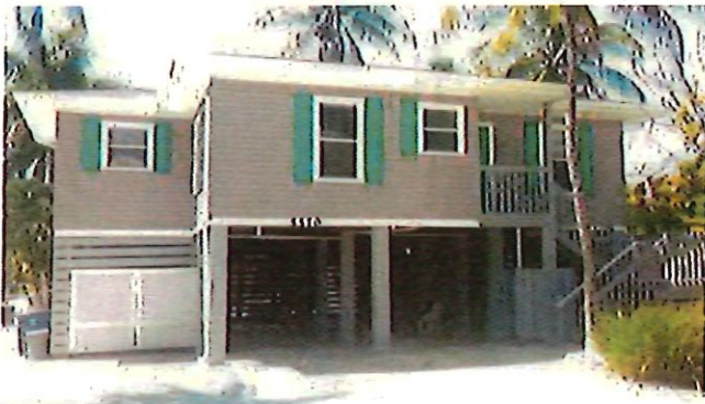
Building Front Photo
