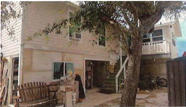
Building Front Photo
