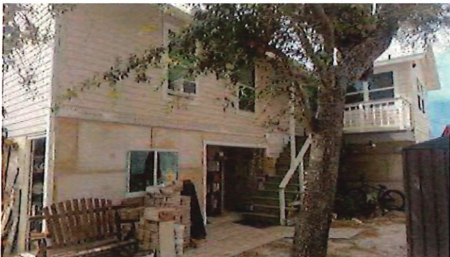
Building Front Photo
