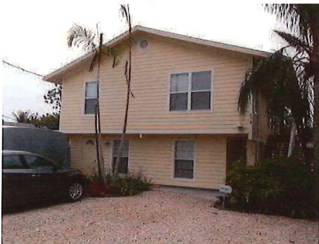
Building Front Photo
