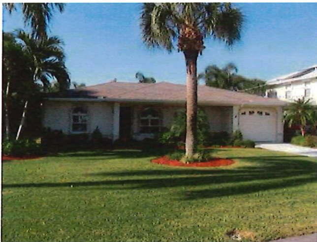
Building Front Photo
