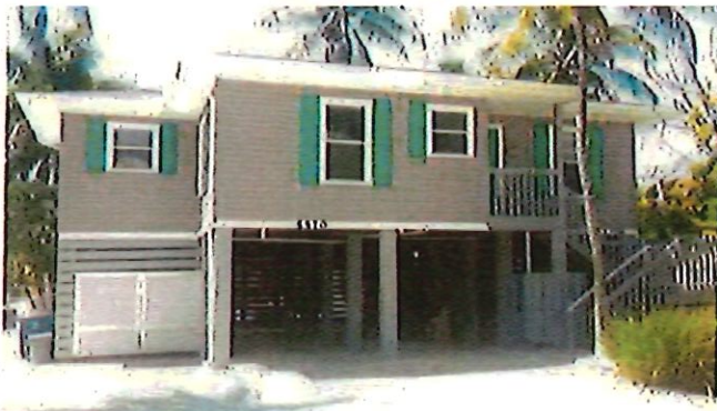
Building Front Photo
