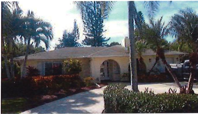
Building Front Photo
