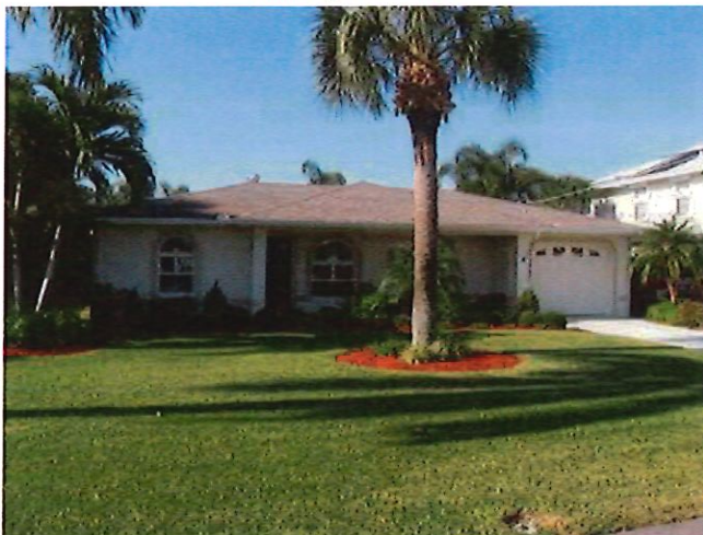
Building Front Photo
