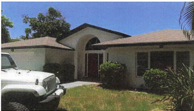
Building Front Photo
