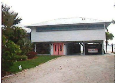
Building Front Photo
