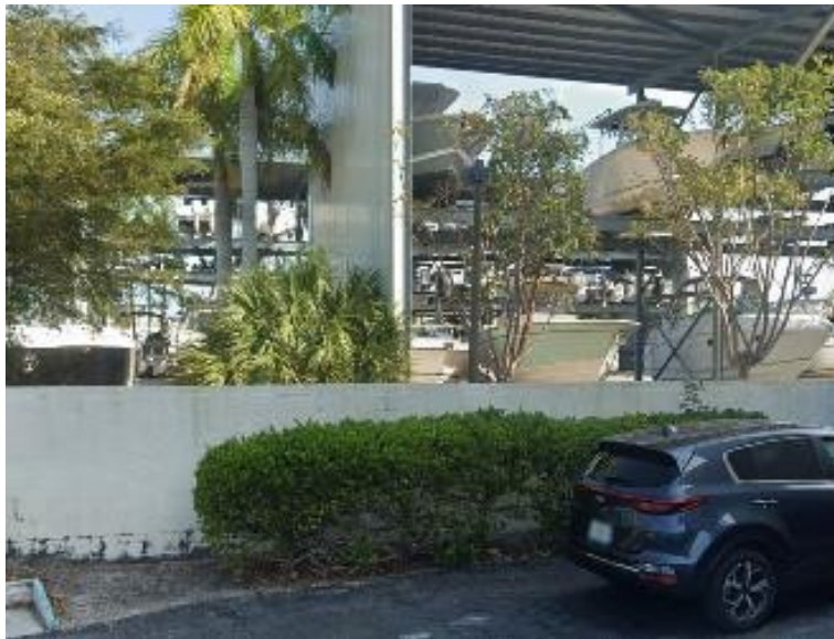
(6' High Wall – pre-hurricane)
