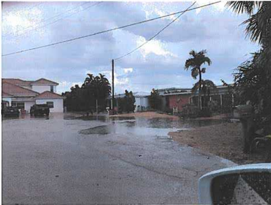
PONDING AFTER WEED BARRIER REMOVAL
