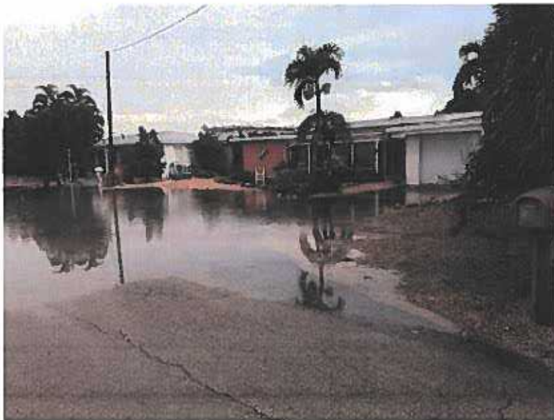
AFTER REMOVAL - WATER HAS NO FORMAL TOWN DRAIN
