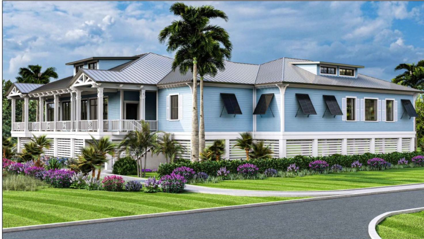
EAST ELEVATION (VIEW FROM STERLING AVE)
