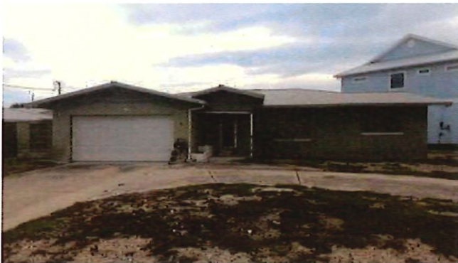
Photo Date: September of 2025
