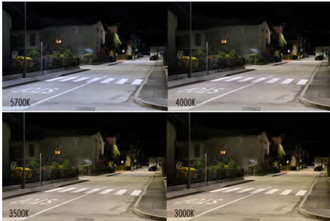
Figure 5 – FDOT streetlight training materials demonstrating the appearance of correlated color temperature (CCT) in Kelvin.
