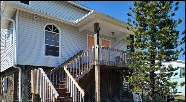
VIEW OF SUBJECT PROPERTY 6036/38 ESTERO BLVD, FORT MYERS, FLORIDA 33931
