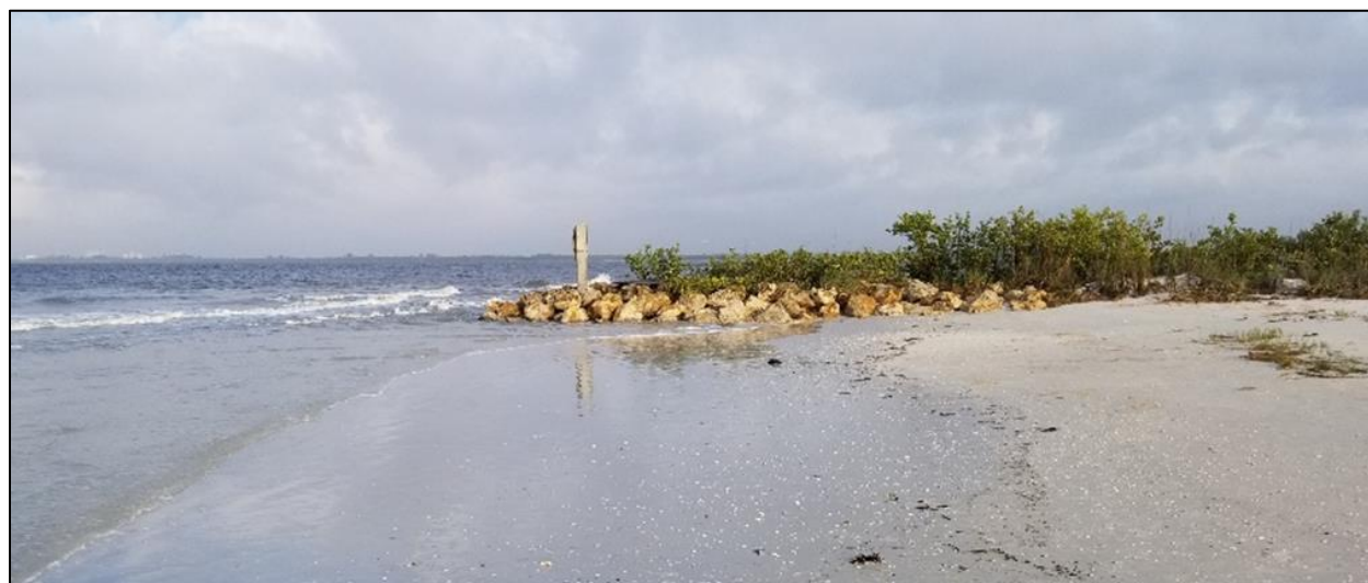
Figure 2. 2011 Project Terminal Groin Located just South of C-174A.
