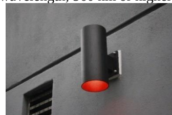
GOOD EXAMPLE: Shielded bulb with Amber LED (long-wavelength, 560 nm or higher)
