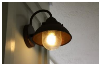
BAD EXAMPLE: Unshielded bulb
